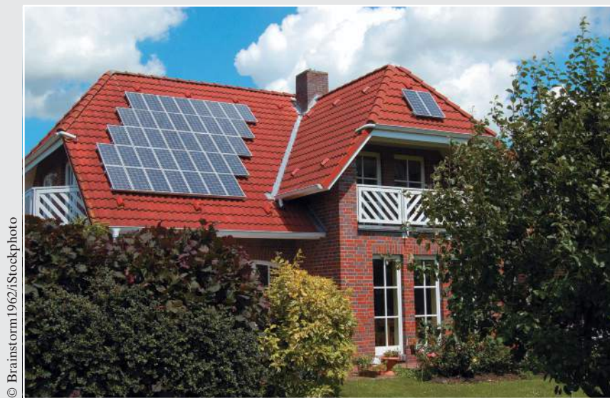
(b) An array of polycrystalline silicon photovoltaic cells.
